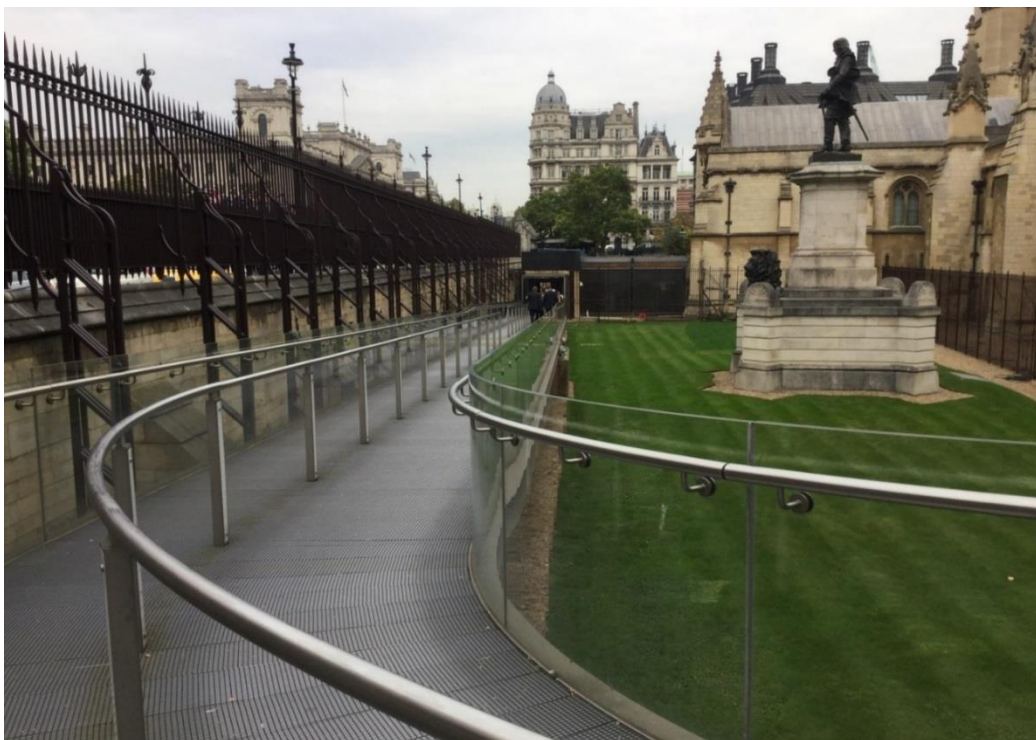
Continuation of the ramp from the Visitor Entrance to the security search point
